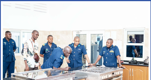
CAS INSPECTING AN EQUIPMENT INSTALLED IN THE OFFICERS' MESS KITCHEN
